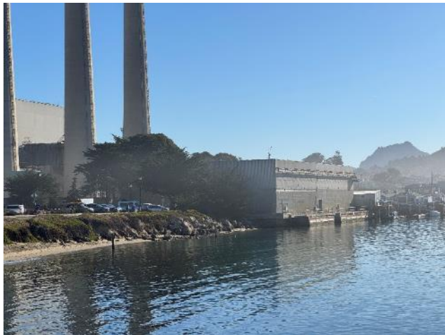
Figure 3.9: Vistra Pump Intake Waterfront Property
