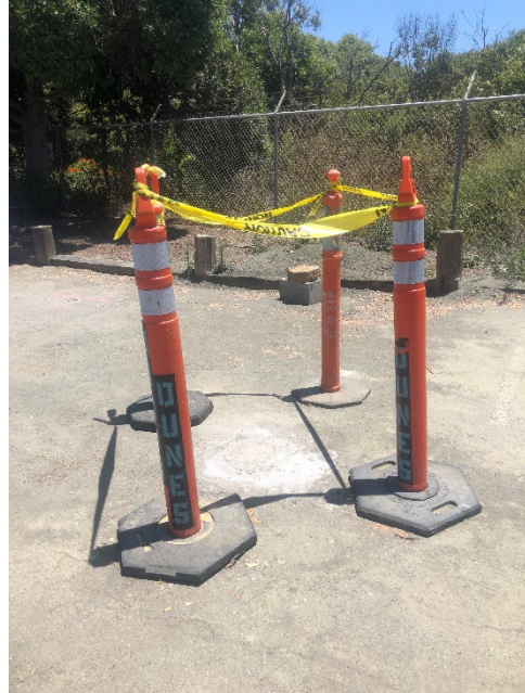
Well Site after Coring and Filling (SB #7)
