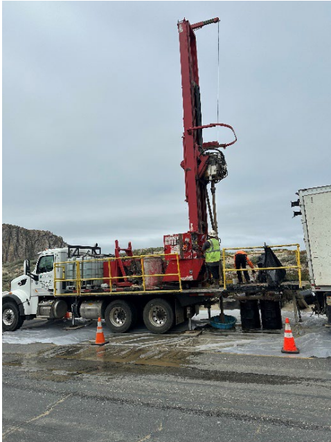
Well Site Coring – Sonic Boring #8 (SB #8)
