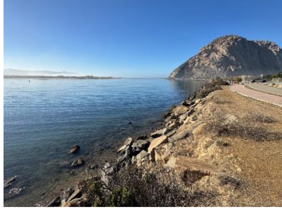
Figure 3.5: Photo of the rock revetment protecting Coleman Park
