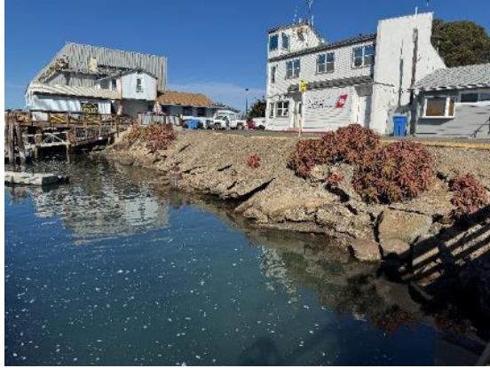
Figure 3.4: Photo of the shoreline protection adjacent to USCG and Harbor Dept.
