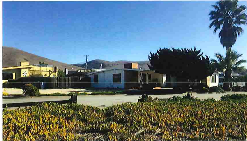
1 (E) RESIDENCE FROM BEACHCOMBER VIEW OF EXISTING CONDITION LOOKING SOUTHEAST FROM BEACHCOMBER DRIVE, SEE IMAGE BELOW FOR PROPOSED DESIGN
