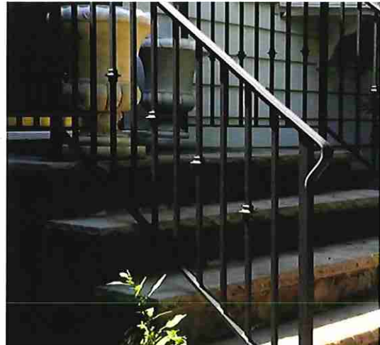
WROUGHT IRON RAILING & GUARDRAILS
